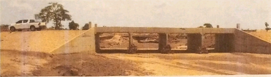
Construction of road infrastructure at Msomera Village.
