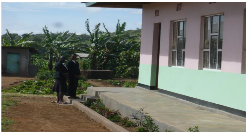
Part of the dormitory/hostel building of CHES
